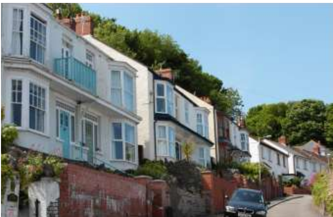
As the slope of Overland Road increases, the views over Swansea Bay influence the designs with bay windows on both floors to benefit from the panorama over Mumbles
